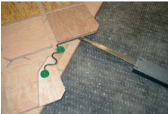
The interlocking system does not only connect adjoining modules, it also ensures a very tight, seamless fit.
